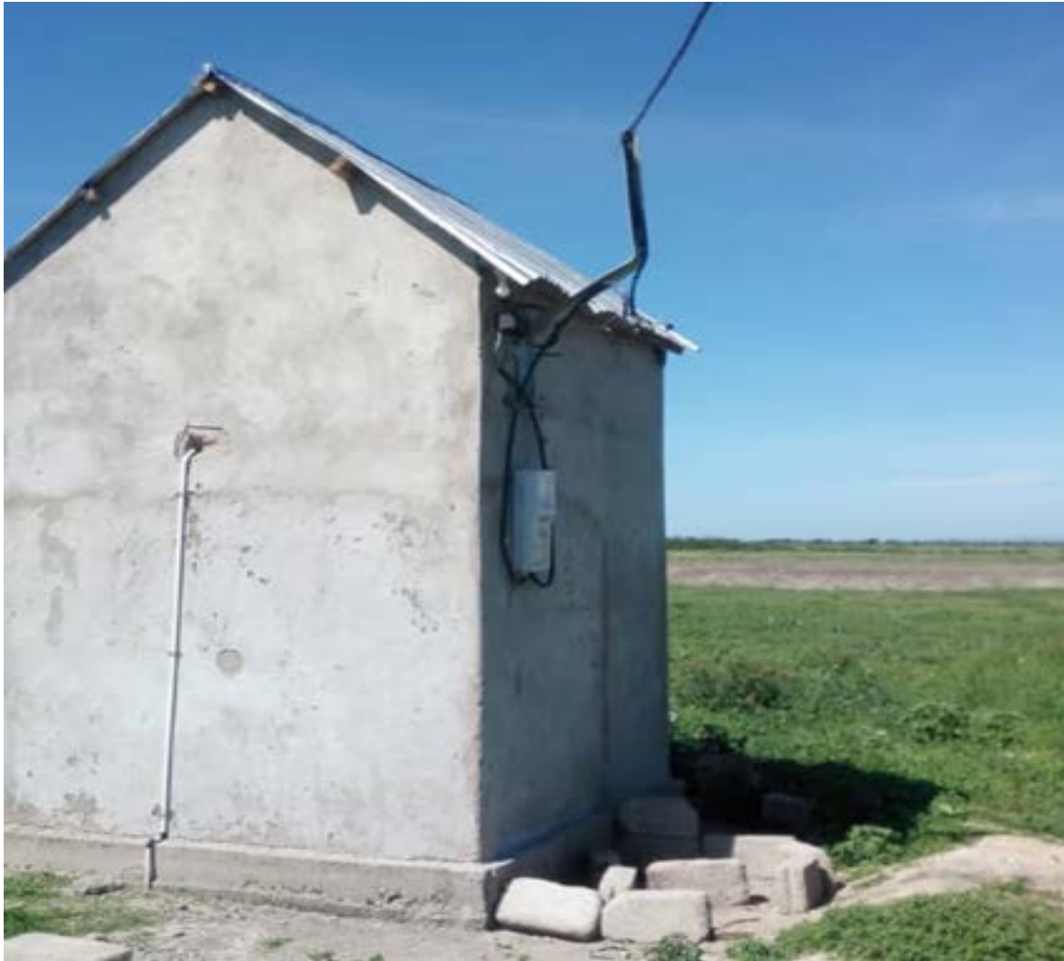
Water Pump House at Nyatwali
